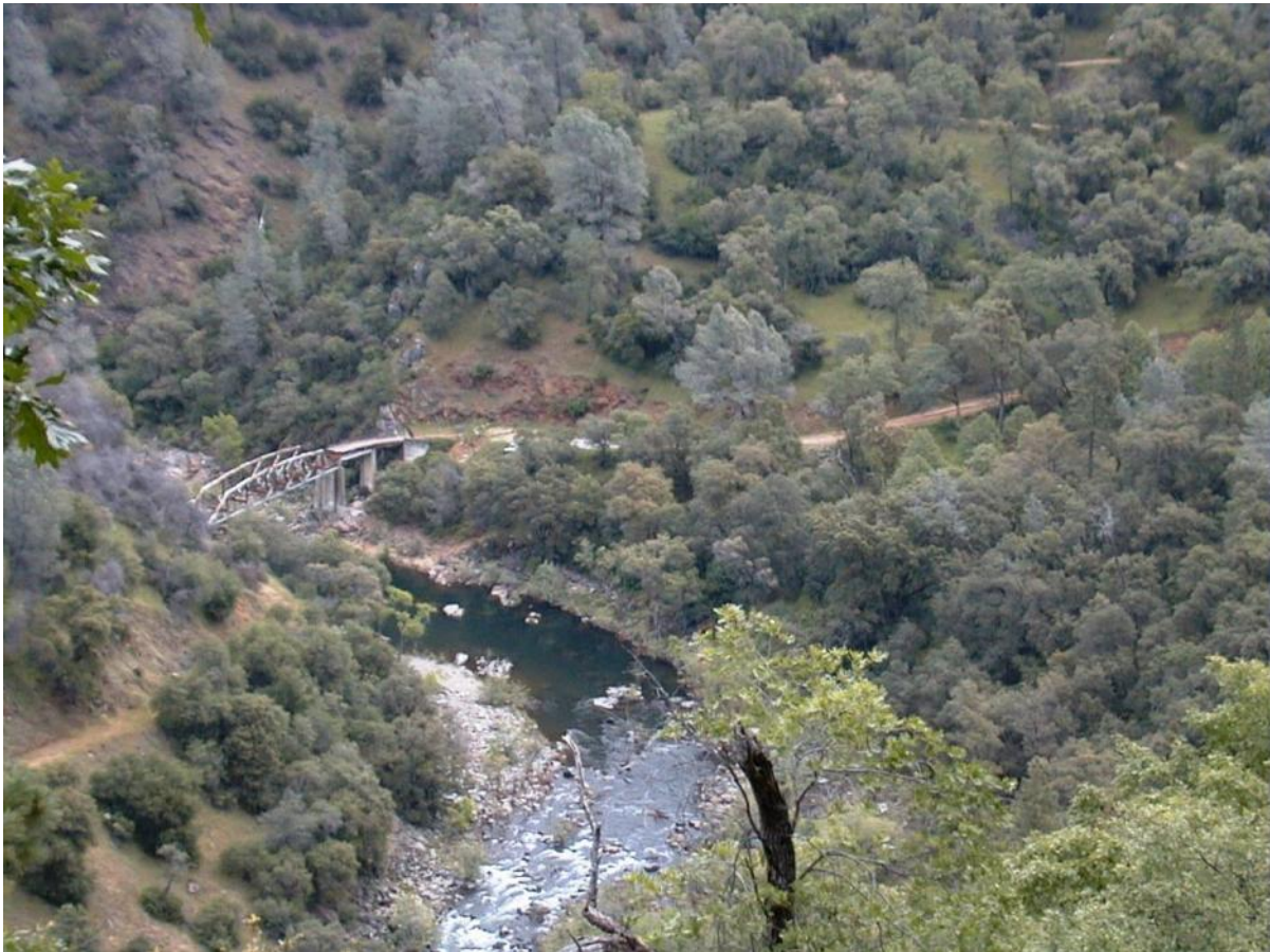
Fig 16. Mokelumne River Bridge on Ponderosa Way over the Main Stem Mokelumne River. Calaveras County is right, Amador is left and PG&E land is middle.
